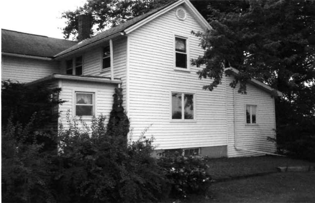
This view is from the northeast corner of the home.
